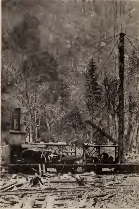
A skidder which brings logs several miles through the air.
